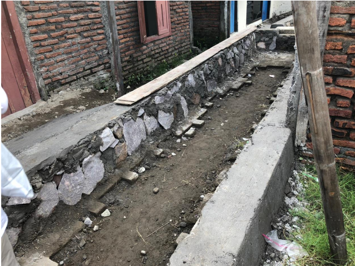
Figure 15: Heightening of the street (van 't Klooster, 2018)
