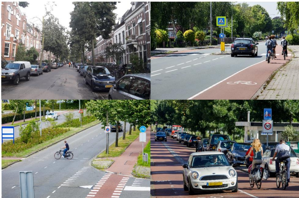
Figure 5.1: Four types of cycling facilities: street without cycling facility (top left) (Van Bergen, 2017); street with marked cycling lane (top right), separated cycling lane (bottom left) and street especially for cyclists (bottom right) (SWOV, 2020).
