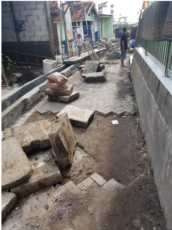
Figure 9: Roadworks in Tambak Lorok
