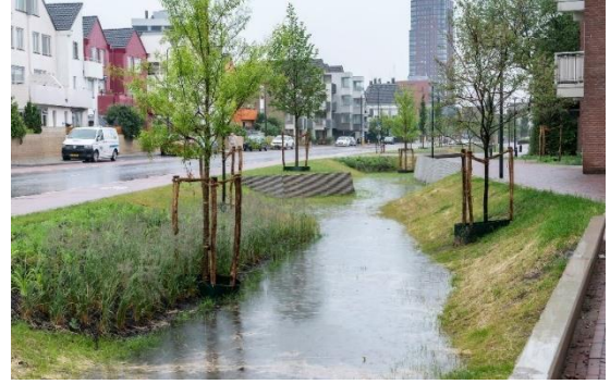
Figure 15: : wadi in Enschede to let rainwater slowly infiltrate into the soil (Gemeente Enschede et al., 2021)
