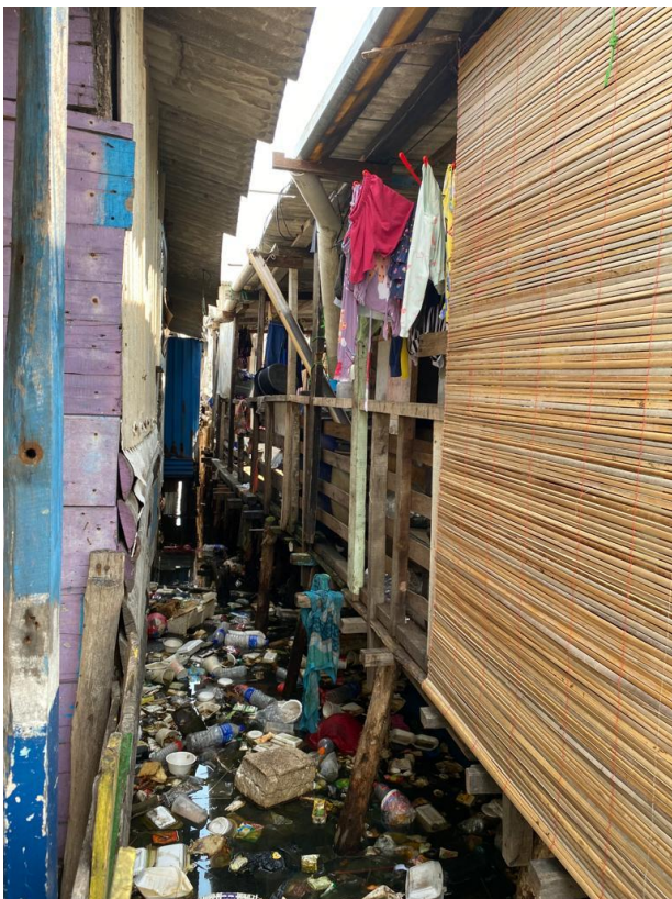
Houses built on stilts in the water in the coastal area
