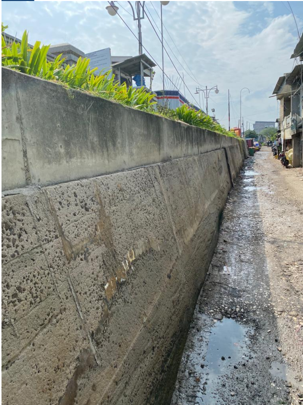
Coastal dike showing the different construction layers developed over the years
