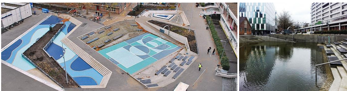
Figure 18&19: Water square Rotterdam Bentheplein during dry and wet conditions (De Urbanisten, 2015)
