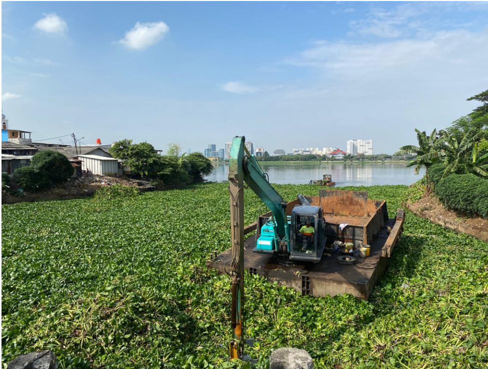
Removal of the water hyacinth by dragging of a water retention area (Waduk) in Jakarta to maintain the storage capacity
