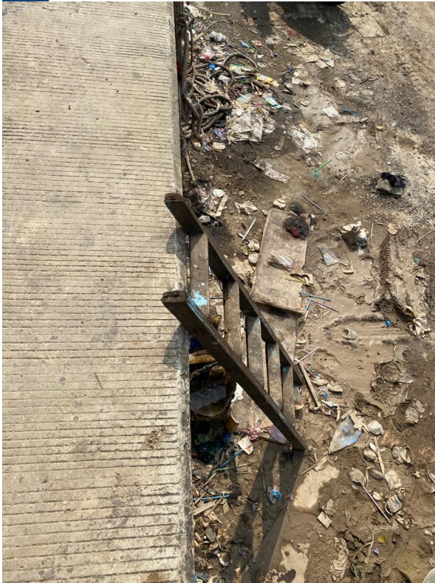
Functionality adjustments made by coastal community to a coastal dike
