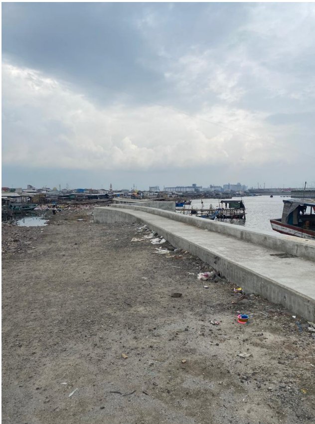
Newly constructed dike section
