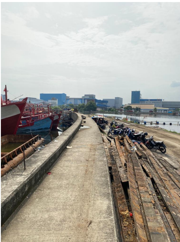
'Regular' coastal dike section
