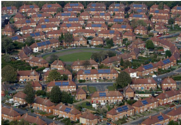
Figure 11 Aspley solar panels
