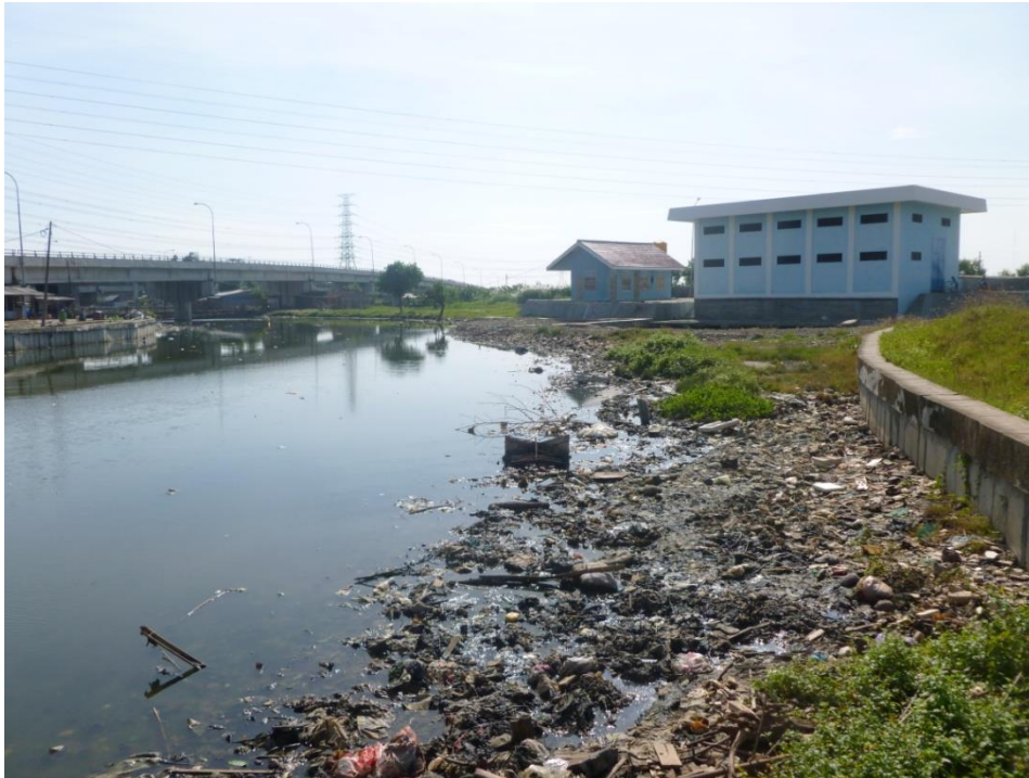
Figure 19: Pump station, polluted river
