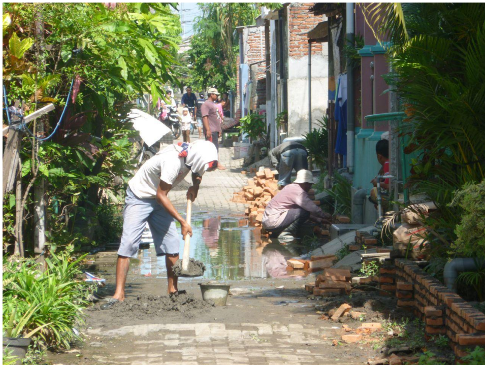
Figure 16: road is getting heightened in Mrs. Sutarni's RT
