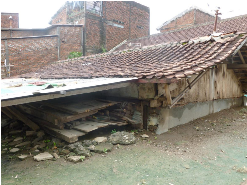
Figure 14: Mr. Sartono's former house
