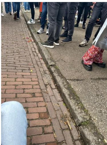
Figure 6 There is no way to get on this curb with this medium-sized wheelchair
