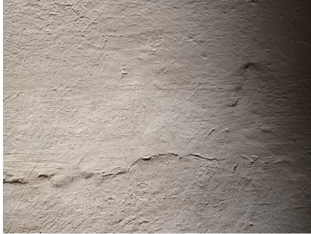
Figure 75: Scratched signs in the wall of a cell in the U-boat
