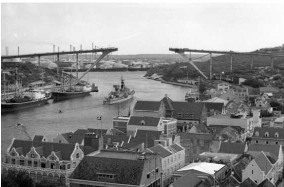
Figure 3.14 – Construction of the Juliana bridge (Makkinga, 2011)
