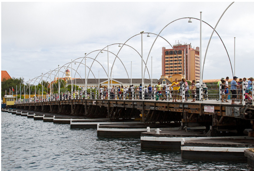
Figure 5.5 – Queen Emma Bridge (De Jong-Lantink, 21-12-2011)
