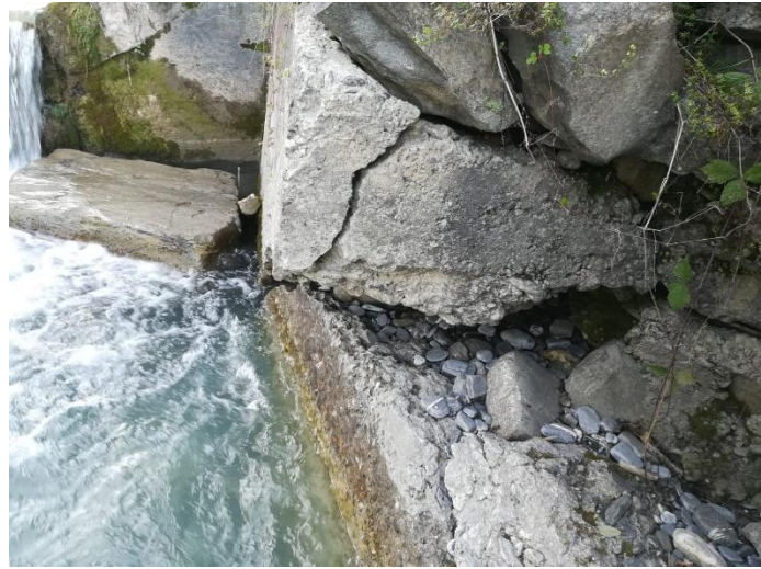
Figure 10: The Effects of Erosion to a Structural Measure near Frutigen (Own Observation, 14-09-2019)
