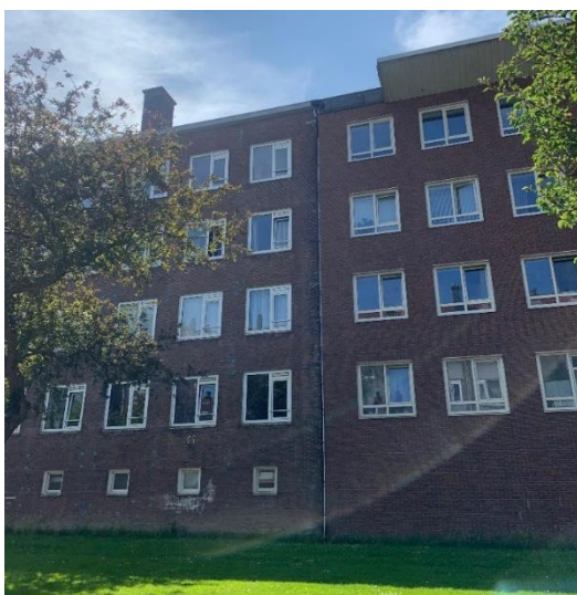
Figure 12: Photo of the partly renovated building Ruychaverkwartier (Own photo, 2025)
