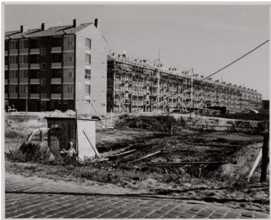
Figure 6: Wildemanbuurt under construction (Amsterdam City Archives, 1959)
