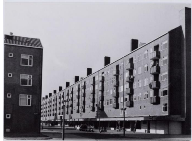
Figure 5: Wegener Sleeswijkbuurt during construction period (Amsterdam City Archives, 1959)
