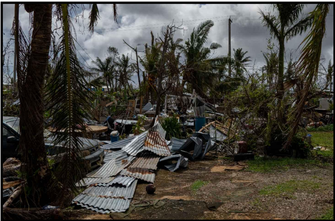
Figure 7. Destruction after Typhoon Mawar, Guam, 2023 (Aguon, 2023).
