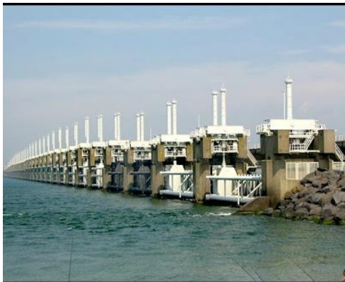
Figure 8: Eastern Scheldt Storm Surge barrier (Rijkswaterstaat, n.d.)
