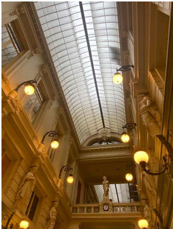
Image 38 - Henri Rieck, Passage du Nord , Brussels, Belgium, 1881-1882. Glass, wood, natural-stone, iron. Image by the author, 2023.
