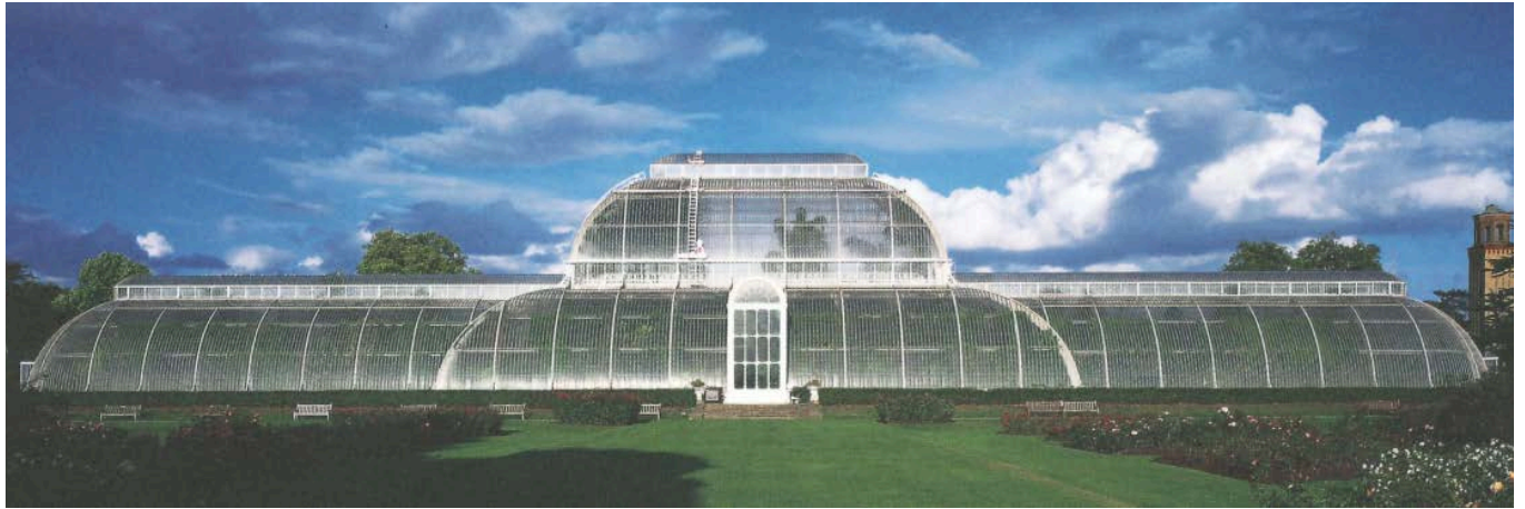
Image 8 - Decimus Burton and Richard Turner, The Palm House at the Royal Botanical Gardens at Kew, London, United Kingdom, 1845-8. Glass, cast-iron. Image from Wigginton, M. Glass in Architecture , London, 1996.
