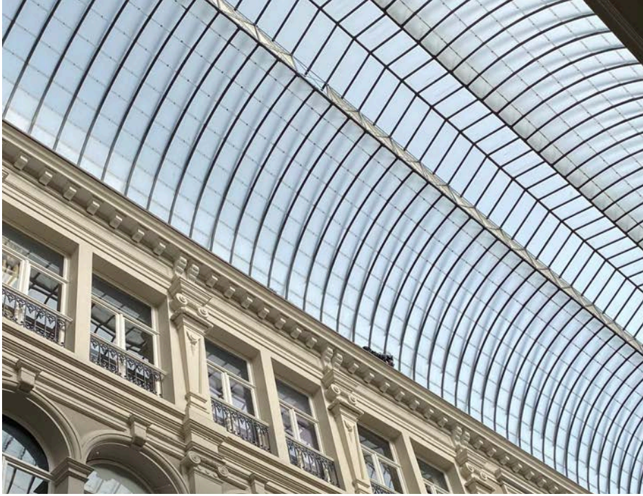
Image 41 - Henri Rieck, (reconstructed) Pyramidal Roof of the Haagse Passage, The Hague, the Netherlands, 1885. Glass, iron. Image by the author.
