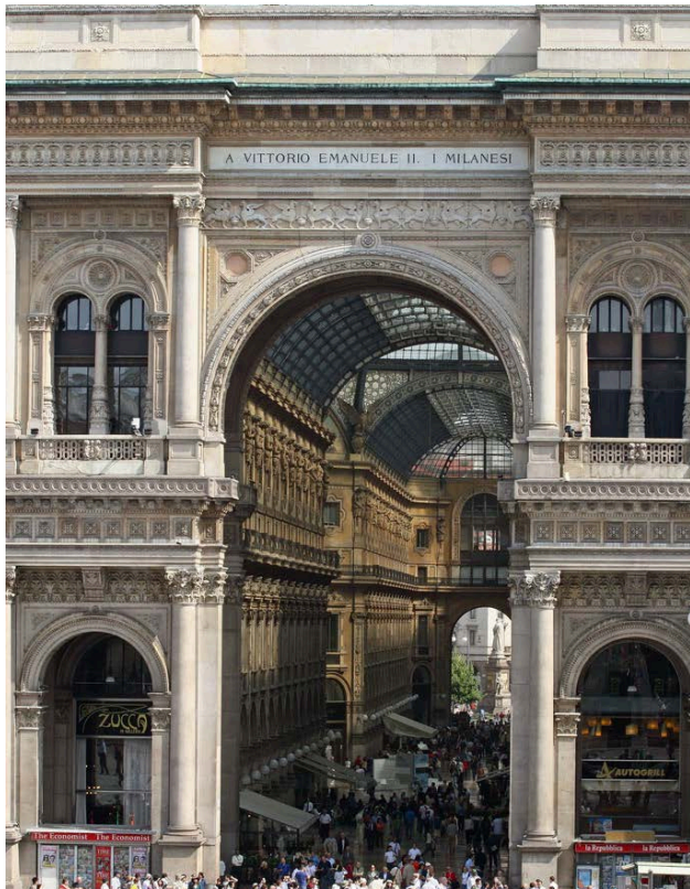
Image 17 - Giuseppe Mengoni, Plan of the Galleria Vittorio Emanuele II, Milan, Italy, 1877. Glass, steel, natural stone. Image by Chris Brown, from https://commons.wikimedia.org/w/index.php?curid=3358948 .
