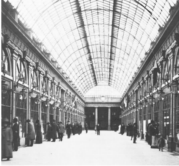
Image 16 - Pierre Fontaine, Passage d'Orléans , Paris, France, 1892. Wood, glass, cast-iron. Image from Geist, J.F. Arcades: The History of a Building Type , Cambridge (MA), 1979.
