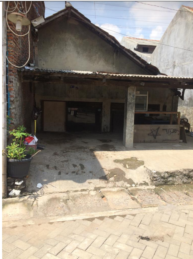
In this picture tilting is visible. But that is not the main problem, that is the sinking part and the fact that the house is flooded.
