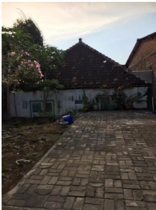
The left part of this house sank further down than the right side. The right side is most likely added.
