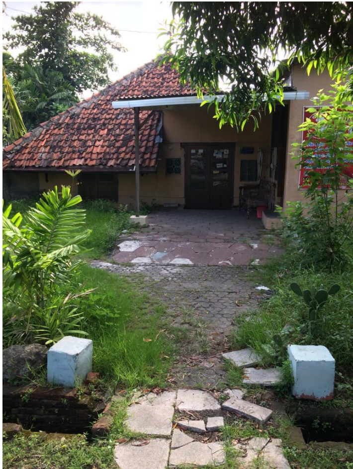
The left part of this house sank further down than the right side. The right side is most likely added.
