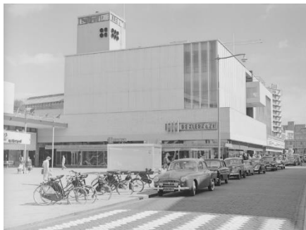
Figure 10. Lijnbaan 150, Rotterdam. De Klerk Building 1956 (Source: wederopbouwrotterdam.nl )
