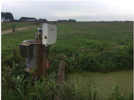
Figure 11: A test location for a pressure drainage system. A well is installed near an open body of water to regulate the groundwater level under a field through a series of pipelines (Own Work, 2018).
