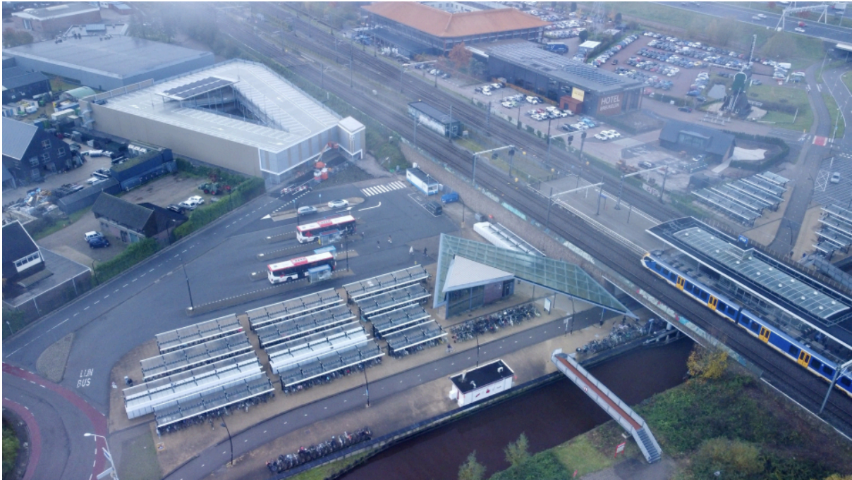
Figure 7: Aerial view of Breukelen station (Provincie Utrecht, 2024)
