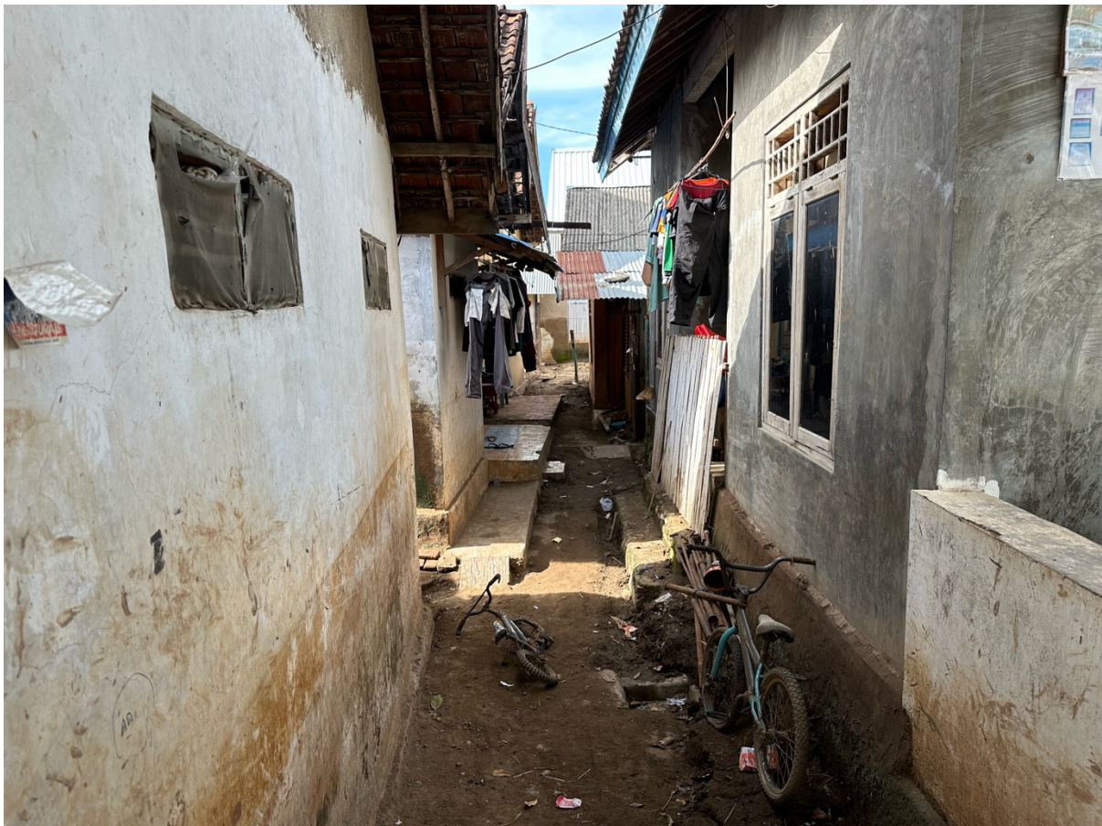
Figure 11: The flood line marked on the houses of Paruga, Bima (by author, 2024)
