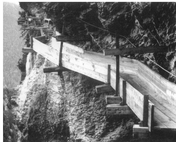
Figure 14, Visualisation aid of construction of bisse channel
