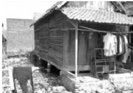
Figure 4.2 – Elevating the house (Marfai & Hizbaron, 2011)
