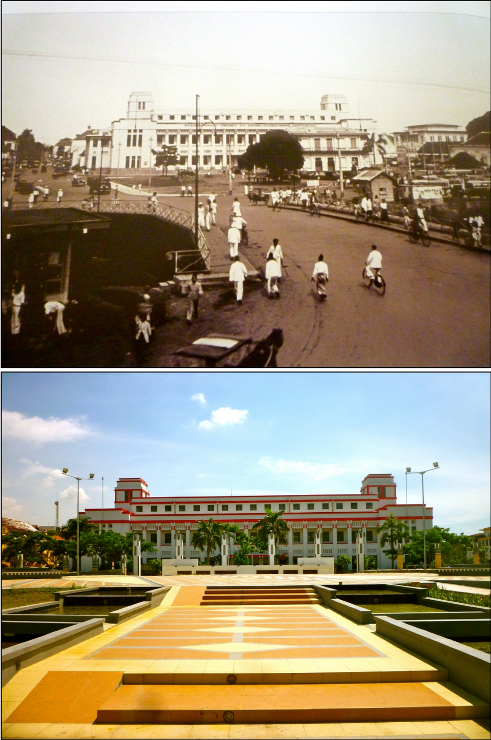
Fig. 4.7 Internatio, view short after completion in 1931 and present. (Source: First photo – Maior, 2004, p. 122. Second photo – Author, 2012)
