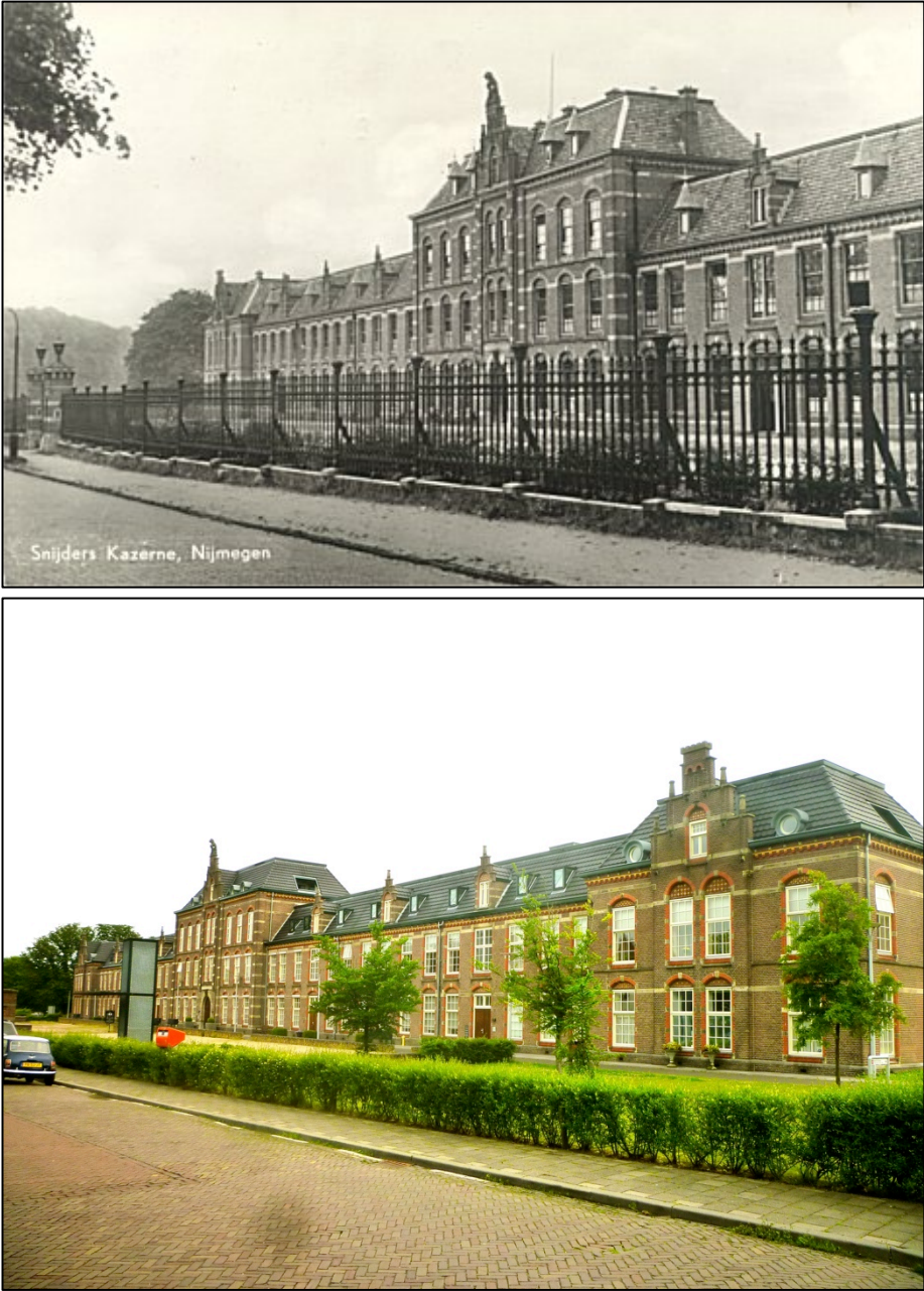
Fig. 4.3 The Snijderskazerne, past and present view. (Source: First photo – Legerplaats, 2011. Second photo – Author, 2012)
