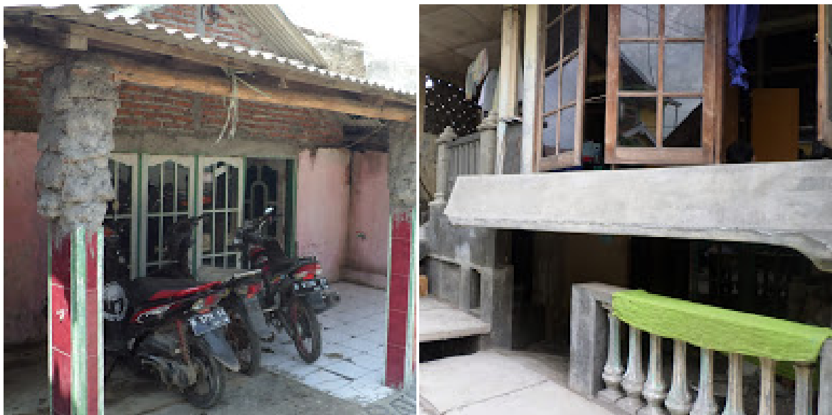
Picture 4 : Heightened sealing (9-1-2014) and Picture 5: Old house sank in the ground (9-12-2013)
